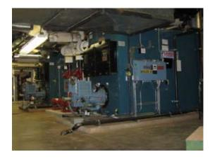
Great example of a baseload system utilizing standard efficiency firebox boilers along with a high efficiency condensing baseload boiler. Condensing boiler shown above circled in red.
