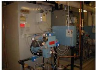
Working with TSP Engineering & Egan Mechanical, Hazelden installed two (2) Bryan RV500 combination gas/oil boilers with input capacities of 5000 MBH. Each boiler was equipped with modulating high turn down Gordon Piatt burners along with Honeywell R7999 Linkageless Fuel/Air Ratio Controllers.
