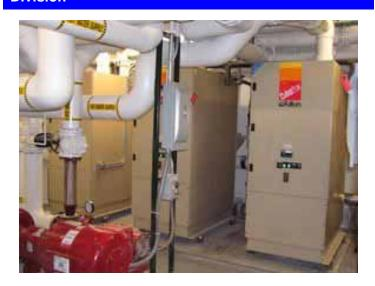
When Seagate's Recording Heads division needed to upgrade their boilers, the Ryan Company was eager to help. We replaced one large firetube firebox boiler at 80% efficiency with three PHW2000 natural gas fired Fulton pulse combustion hot water boilers. Each Fulton boiler has an input of 2,000,000 BTU/HR and is equipped with modulation which produces efficiencies up to 98%.
