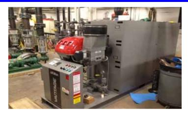
Located in Fargo, North Dakota Mechanical Engineer: Obermiller Nelson Engineering Mechanical Contractor: Peterson Mechanical Inc. Equipment: -(2) Fulton Vantage Condensing Boilers - Model VTG2000 DF -Dual Fuel Burners: Natural Gas and Fuel Oil #2 -Each Boiler is 2000 MBH input. -Fulton ModSync Sequencing Controller
