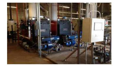
Located in Red Wing, Minnesota Mechanical Engineer: Dolejs Associates Inc. Mechanical Contractor: Ryan Mechanical Equipment: -(2) Aldrich Horizontal Fire Tube Steam Boilers - Model A3S-4040-GO -Dual Fuel Power Flame Burne: Natural Gas and Fuel Oil #2 -(1) Shipco Blowdown Separator
